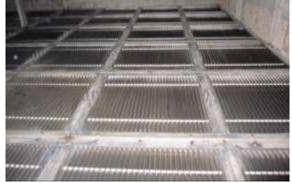
Fig. 7: W-type water-retaining plate group.
