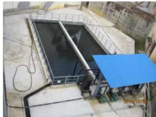
Fig. 9: Recirculation pool after 1 week.
