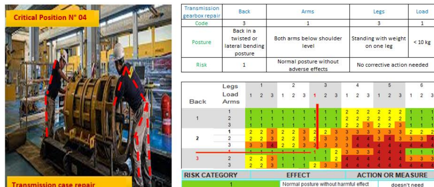
Fig. 5: Critical Position 4 "Transmission Case Repair"
