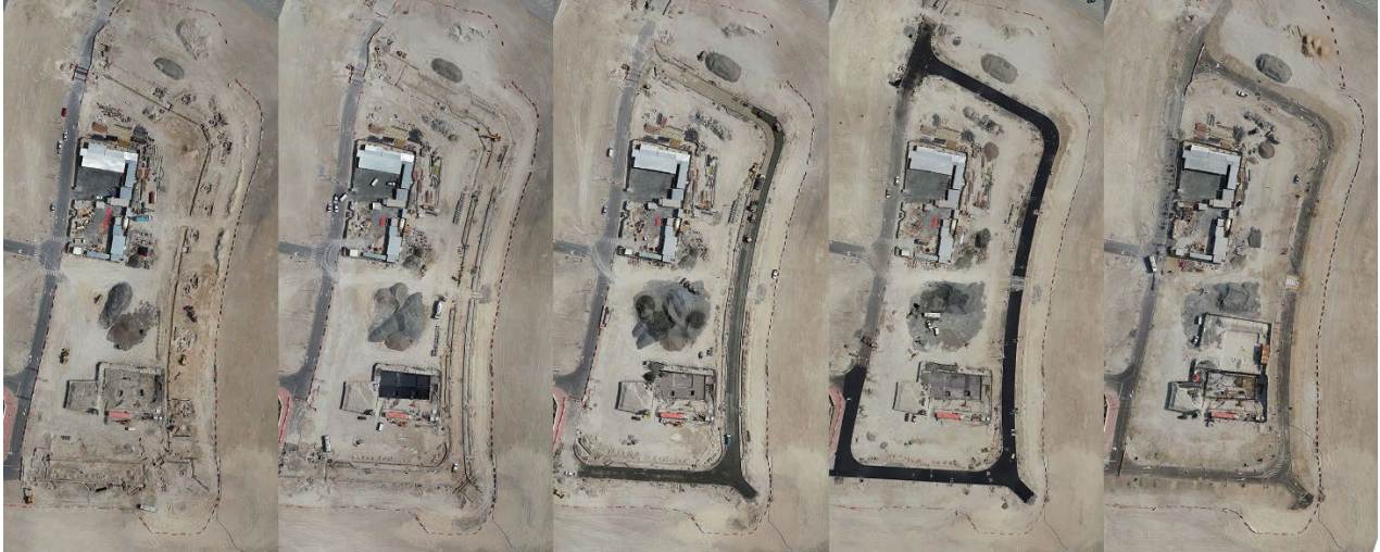
Figure 6. Example of subcontractor progress monitoring using drone technology in road construction [17].
