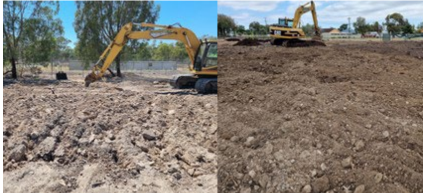
Plate 4: Deep ripping of trial plots to aerate soil and remove compaction.
