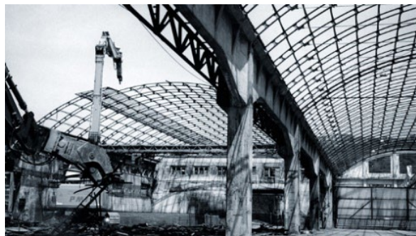
Fig. 3 Dismantling and demolition phase of the roofs [3]
