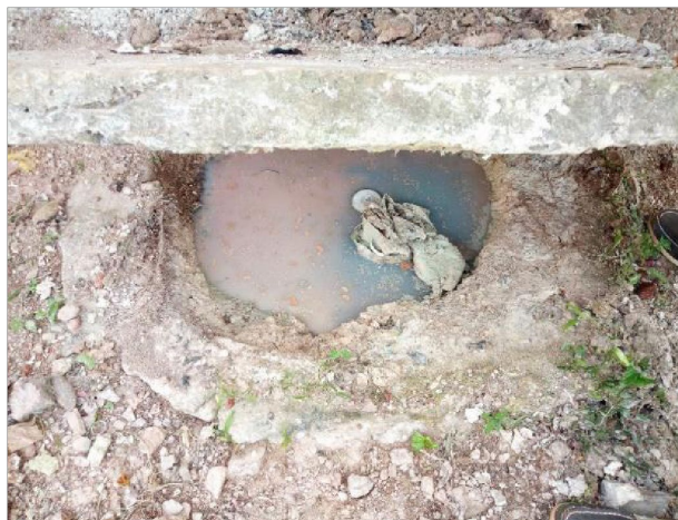
Fig 1: Showing the underground pit
